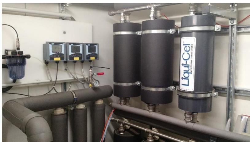
Figure 1.19 – Small scale biogas upgrading unit using hollow fiber membrane contactors
