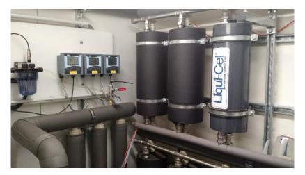
Figure 1.19 – Small scale biogas upgrading unit using hollow fiber membrane contactors *Plant capacity:*  $6 Nm_{CH_a}^3 \cdot h^{-1}$  - *Germany*
