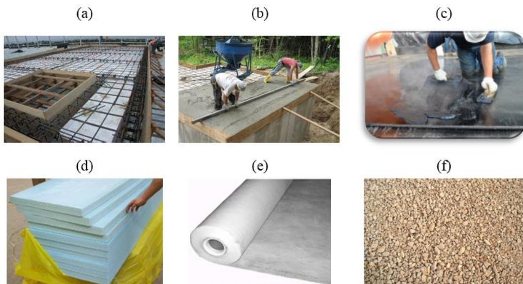
Figure 1-2: TGBR components: (a & b) roof assembly (c) mastic asphalt (d) thermal insulation boards (e) filter sheet (f) pebbles
