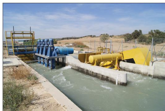
**Photo 5.** The semi-arid Ebro valley concentrates the largest irrigated areas in the basin, supplied by an extensive network of reservoirs and canals. Left: the *Bardenas* canal ( $60 \text{ m}^3/\text{s}$ ). Right: the *Aragon y Catalunya* canal ( $36 \text{ m}^3/\text{s}$ ) is a reversible irrigation canal supplying water from the *Sotonera* or the *Grado* dam, depending on reservoir levels. (Sept. 2013)
