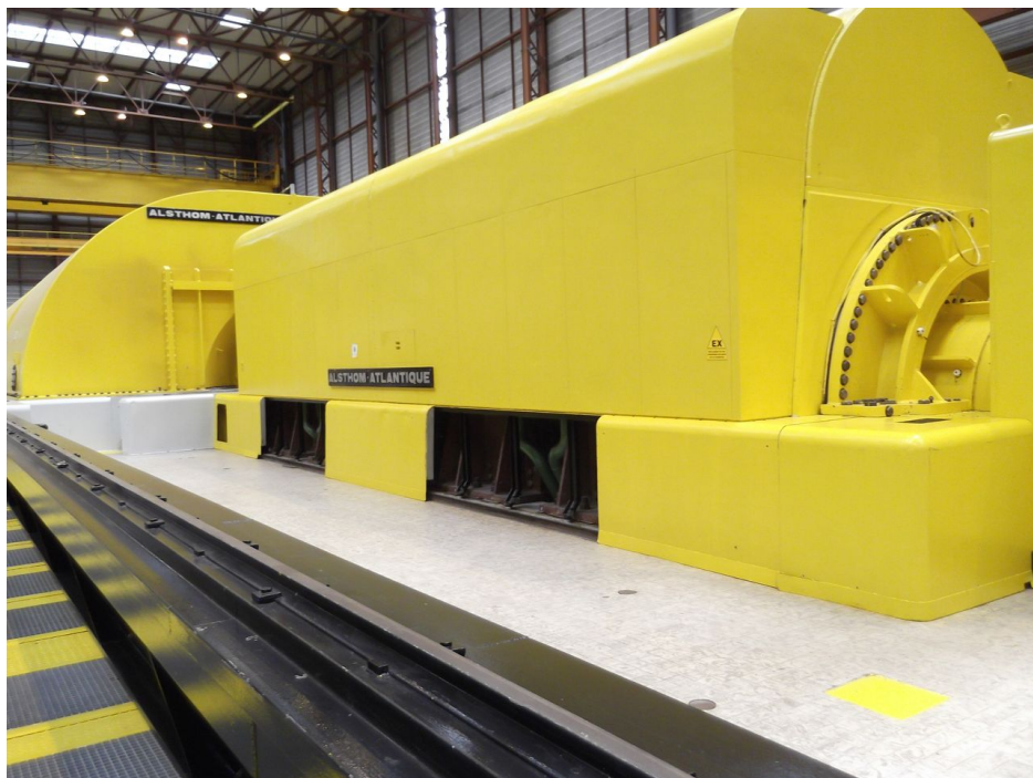
Figure 5.4.: A power plant turbo generator for the generation of electric power
