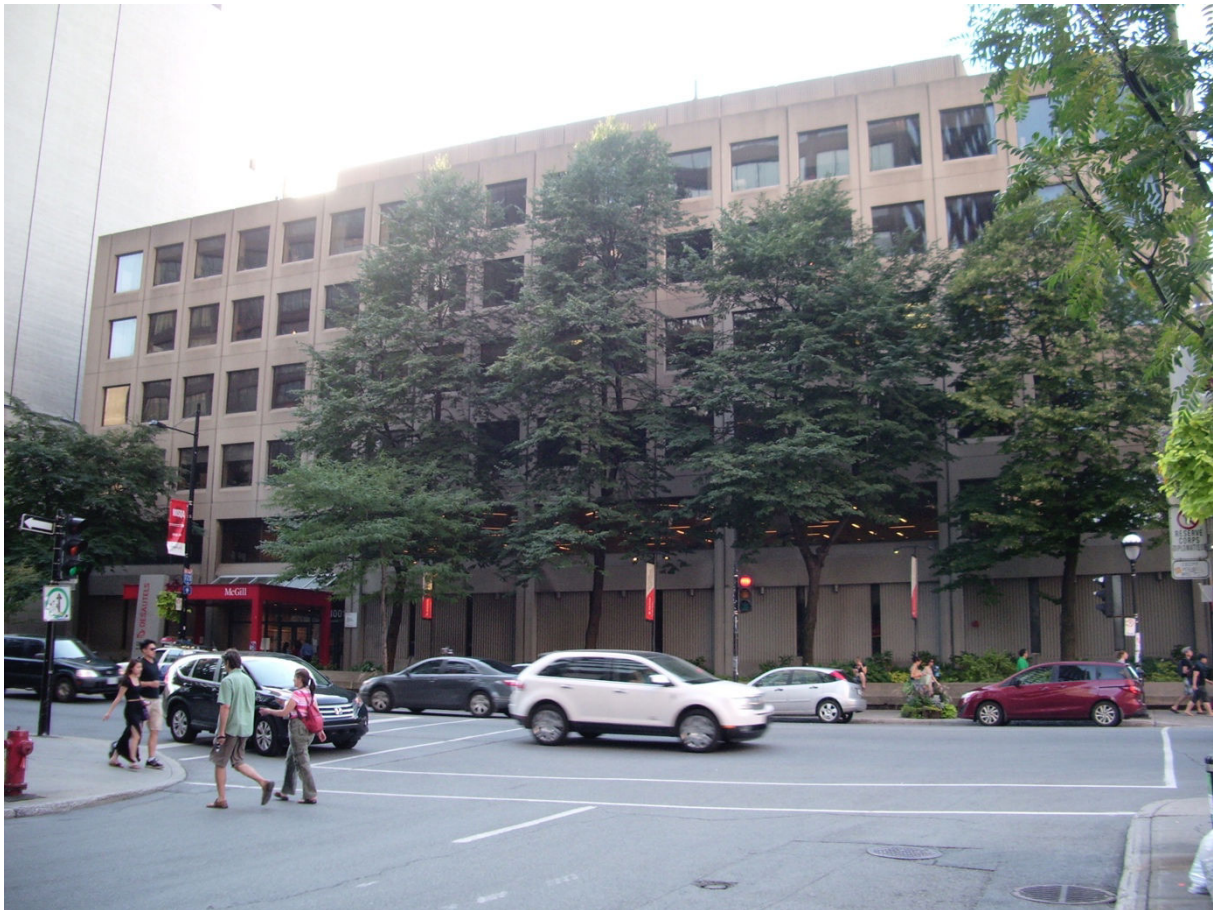
Figure 8 – The Bronfman Building, Sherbrooke Street, Montreal (Canada) (Author)
