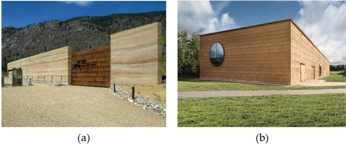
FIGURE 1.1: Rammed earth construction in the world; (a): The Nk'Mip Desert Cultural Centre in Canada [Tri10], (b): Herb Center in Switzerland [Ric14]
