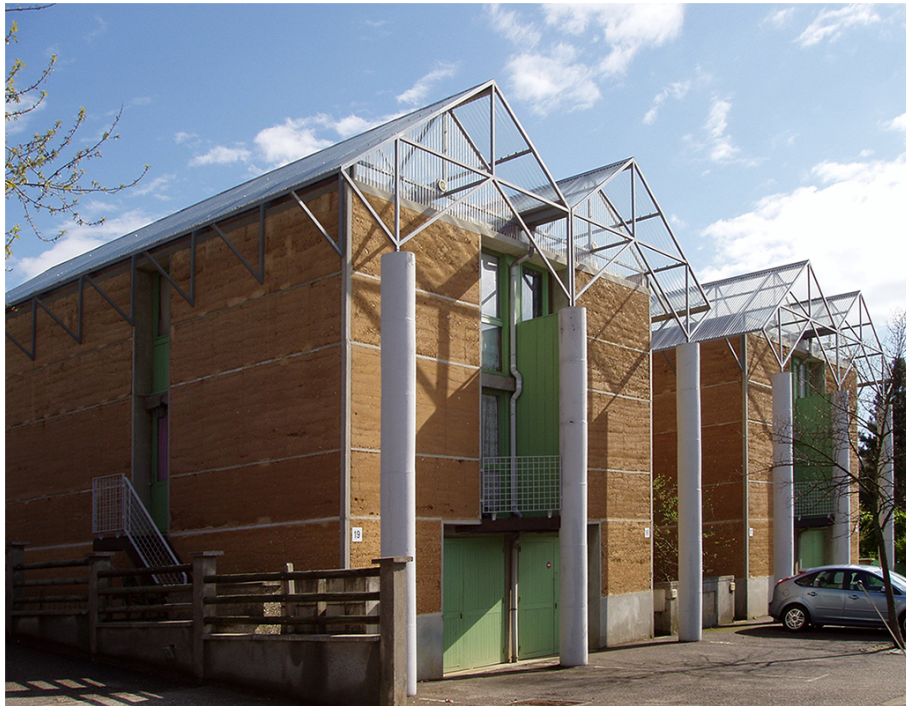
FIGURE 1.3: Social housing in the district of l'Isle d'Abeau-Rhône in France [Aur14]
