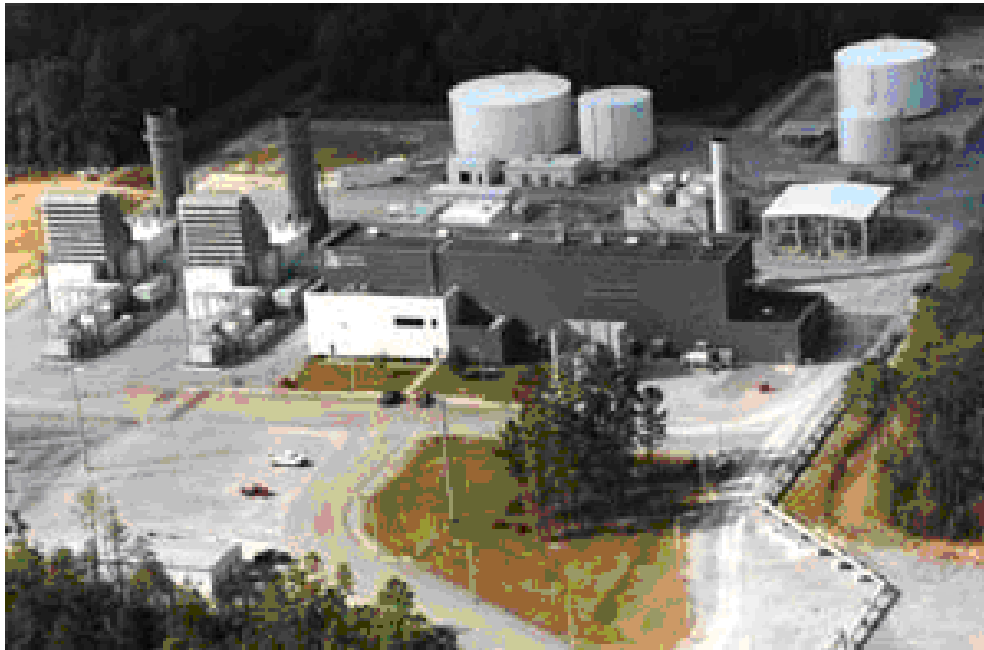
Fig.1.5 Huntorf CAES power plant in Germany
