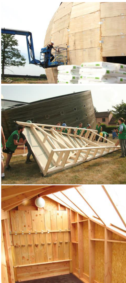
Figure 139. Top. Plywood used as structural material for the Solar Energy House project (see section 5.5). Middle. Moisture-resistant particle board used as roof sheathing at the wood challenges 2015. Bottom. OSB panels used as wall sheathing at the wood challenges 2016. Photos O.G.
