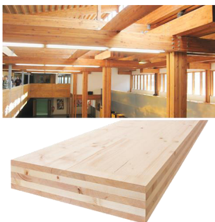
Figure 138. Top . Glulam beams. Vincent Van Gogh High School by Cartignies-Canonica architects, 2006, Blénod-lès-Pont-à-Mousson – France. Bottom . A CLT panel.
