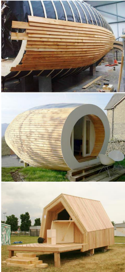
Figure 144. Top. English cedar siding is curved following the pod's geometry. Middle. The Glam Pod in its finished state. On gaukrogerandpartners.com Bottom. Cabin (tiny house) designed and built by students at the wood challenges ( Défis du bois ). Photo O.G
