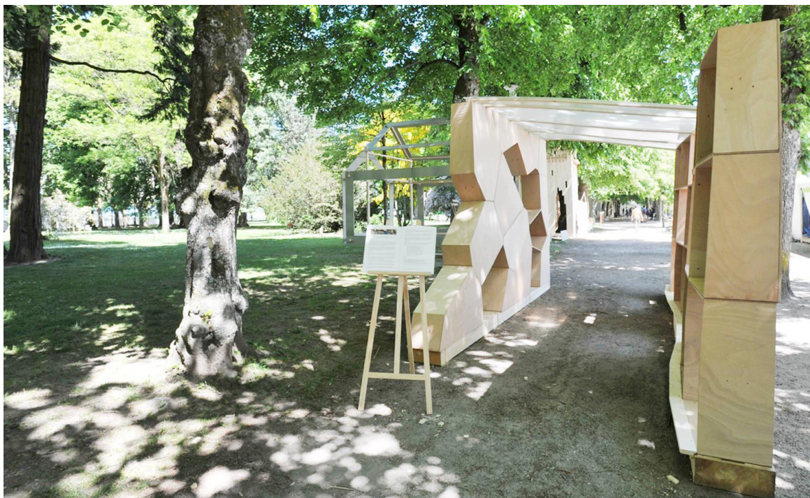
Figure 184. Finished prototypes validating Fab-Cell's first version functional span.
