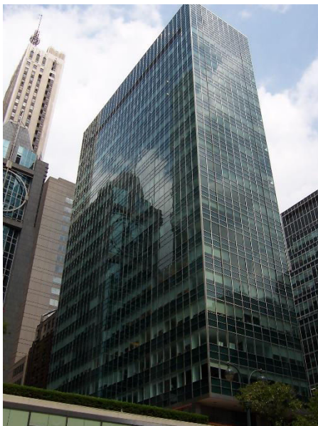
Figure 21. International Style. Lever House Building by Gordon Bunshaft, 1952. On: michaelminn.net
