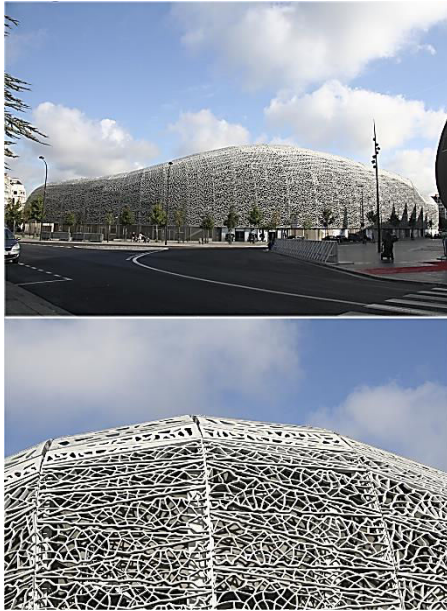
Figure 61. Façade panels derived from a digitally-made biologic-like pattern. Two types of pattern are repeated and adapted over a manifold set of panels whose dimensions change in function of the stadium's geometry. Paris Rugby Stadium at Boulogne-Billancourt, by Rudy Ricciotti. 2007. Photo O.GAMEZ
