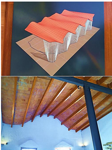
Figure 55. Waved walls and roofs at the Sagrada Familia school. Standard monads (bricks) are used to build these Non-Euclidean bodies. Although regular monads are used for its construction; a specific placing technique and joint distance variation allow for the achievement of form. Notice that special formwork was needed as well. Antoni Gaudi, 1907. Photo O.GÁMEZ
