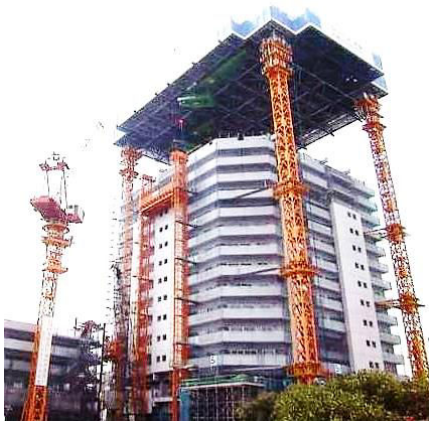
Figure 98. BIG CANOPY. A system for erecting buildings in full automation mode. The canopy has a set of manipulators that perform construction operations. As floors are finished, the canopy will then add another section to the vertical displacement rails as to keep climbing up. Obayashi Corp. 1995. For more information please refer to (Wakisaka et al., 1997). Image On: www.obayashi.co.jp
