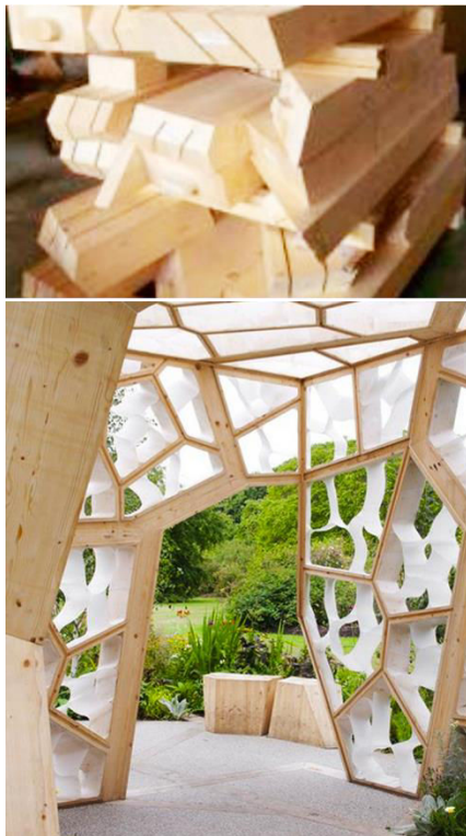
Figure 149. Top. Timber structural members. Observe the complex geometries yielded as result of carving joinery on workpieces. Bottom. Interior view. Observe how structural items are jointed at manifold intersecting angles. Top image (Blumer Lehmann, 2012), bottom image (Nex Architecture, 2011)
