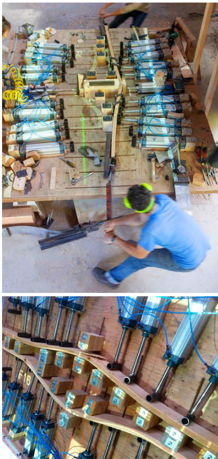
Figure 112. Timber Seasoning Shelter Project. AA, London - Hooke Park. 2014. Structural beech members being bent after undergoing steam softening. Top. Workpiece placed over a template before forming. Bottom. Pneumatic jacks making pressure over workpieces to give them the desired shape. Some planks break,. Some others perform as needed.
