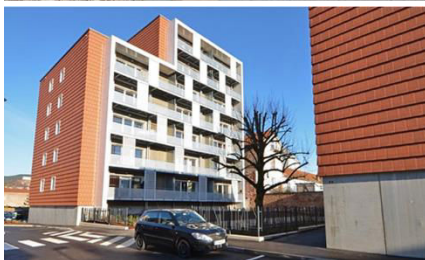
Figure 156. Top. Façade envelope straw-bale-filled insulating unit (cassette). Bottom. Jules Ferry Dwellings. Image credits. Top-J.C Bignon, Bottom (Pagnoux, 2014)
