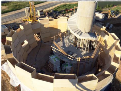
Figure 151. Solar Energy House. Top. Structural members staggered. Notice that the roof rests over the cassette-made enclosing wall. Middle. Closing wall variable section. Bottom. Aerial view of the structure's mounting process. Notice that timber cassettes are installed empty. Insulating material was blown-in once the mounting was finished. Image credits. Top, O.G; Middle, Cartignies-Canonica architects; Bottom, charpentres-bois.com
