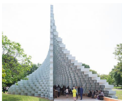
Figure 82. Brick-like patterned structures for the Serpentine Pavilion 2016. Monads are brick-like fiberglass cassettes whose depth varies in function of a horizontal progressive displacement. All cassettes form two grid-like walls sharing the pavilion's structural stability as they are supported on each other. 2016, BIG architects. London, England.
