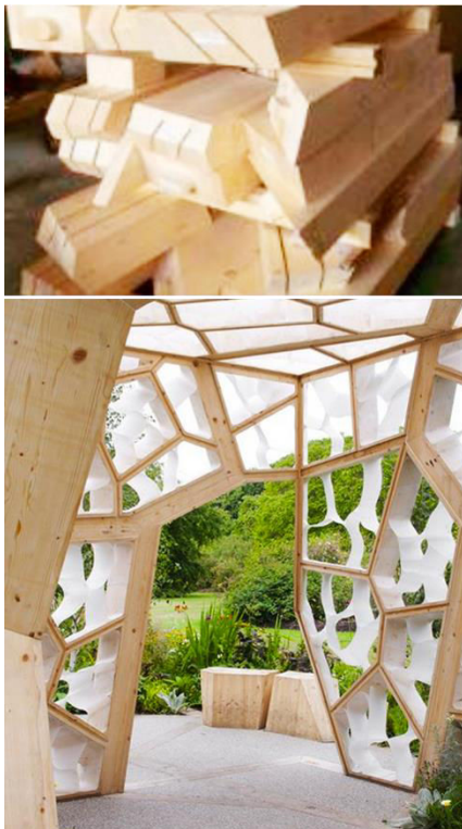
Figure 149. Top. Timber structural members. Observe the complex geometries yielded as result of carving joinery on workpieces. Bottom. Interior view. Observe how structural items are jointed at manifold intersecting angles. Top image (Blumer Lehmann, 2012), bottom image (Nex Architecture, 2011)
