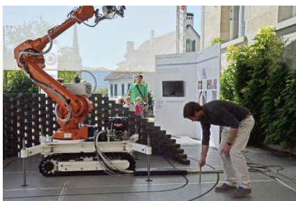
Figure 114. In-Situ robotic fabrication project by V.Helm (2014). A robot builds a non-standard brick wall, by recognizing (through sensors) a drawn path. Image on: http://gramaziokohler.arch.ethz.ch
