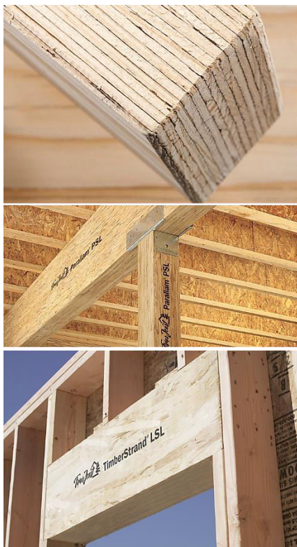
Figure 137. From top to bottom . LVL, PSL and LSL wood composites. On: woodhavenlumber.com & materia.nl.
