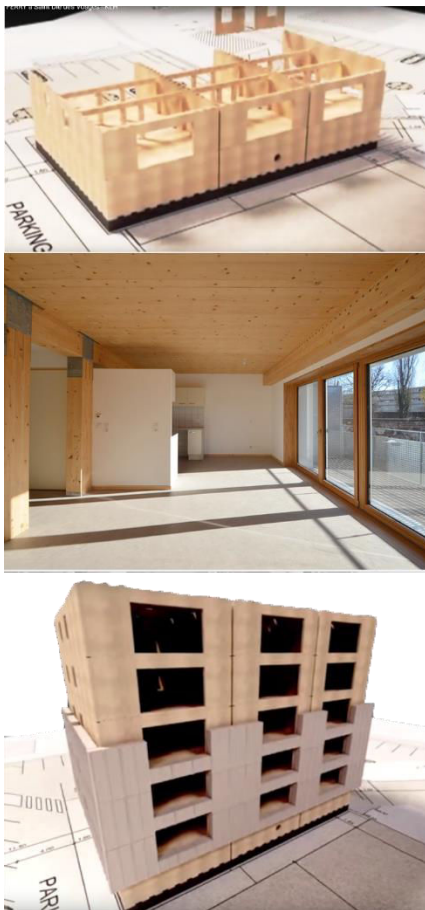
Figure 155. Top. CLT structure. Walls, beams and columns. Middle. Interior finish given by timber panels. Bottom. Timber cassettes as insulating envelope. Image credits. (KLH LIGNATEC, 2013; Pagnoux, 2014)
