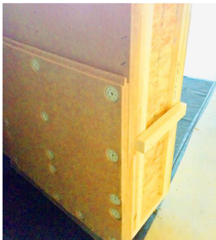
Figure 154. Top. BIM model including carpentry data. Bottom. Wall curvature second solution by full-scale prototyping. A 2x10 mm OSB sheathing replaces 18 mm sheathing for achieving a smoother bending and avoid breaking. Top image courtesy of Dform architecture. Bottom image J.M.
