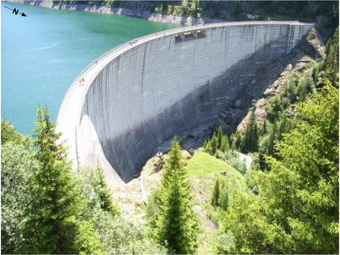
FIGURE 2.6: Double curvature, 69 m high and 250 m long arch dam in Saint Guérin.
