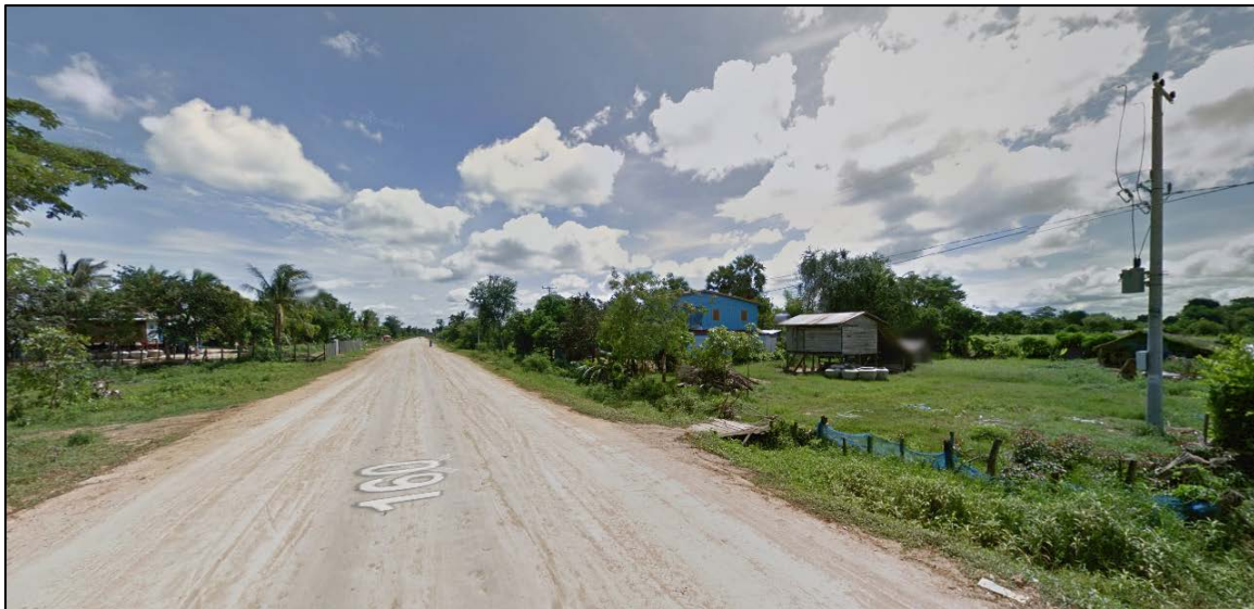
Figure III- 1 : Low-voltage distribution system in Bavel-Battambang-Cambodia [13°18'28.8"N,102°52'54.4"E]
