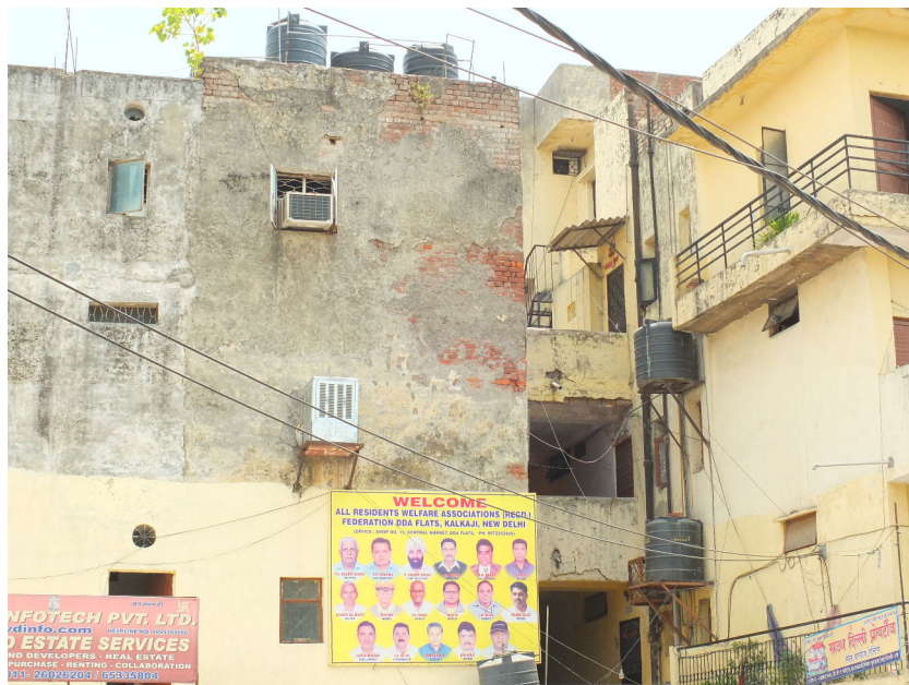
FIGURE 12 – Citernes à Govindpuri (Delhi) (photo : Somsakun Maneerat, 2013)
