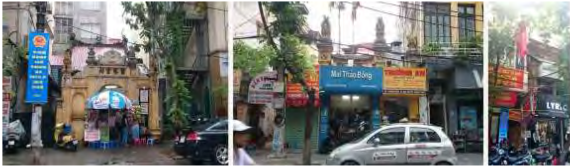
Figure 4.14. Encroachments on some temples: An unnamed temple on Ba Trieu street, Temple Vong Tien and Thien Tien on Hang Bong street and Temple Hoa Than 27 on Hang Dieu street [Photos: Dao Thi Nhu, 2016]
