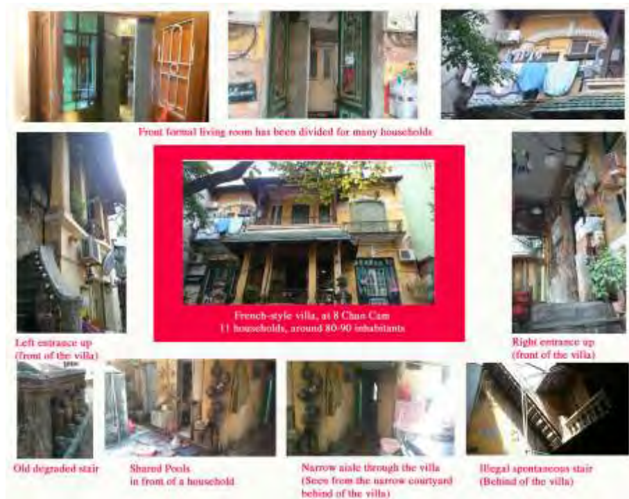
Figure 4.18. Degraded villa at Chan Cam street [Photos: Dao Thi Nhu, 2016]
