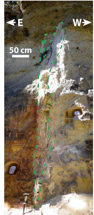
A2. Outcrop view of the site of Saint Michel. The cluster formed in strike-slip regime and is visible exclusively out of shear plane.
