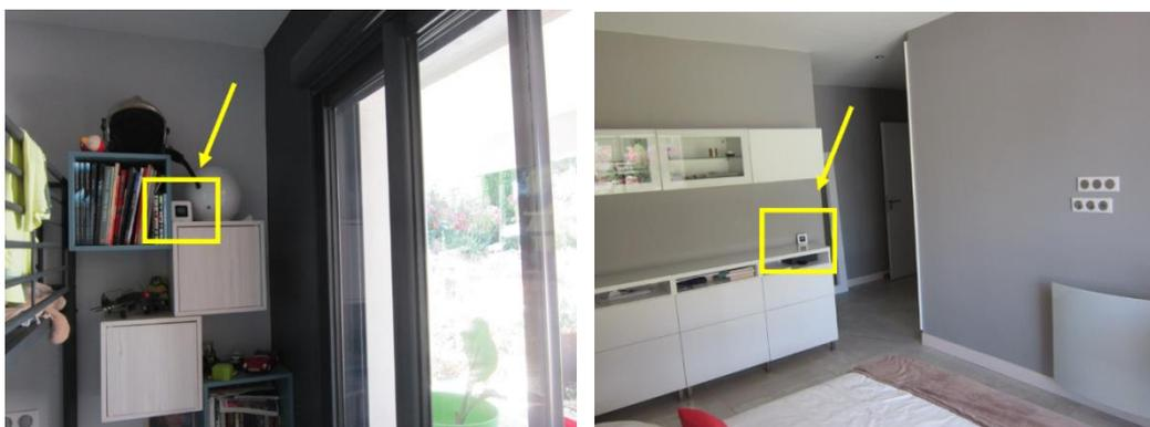
**Figure 4-14: Indoor temperature sensors**
