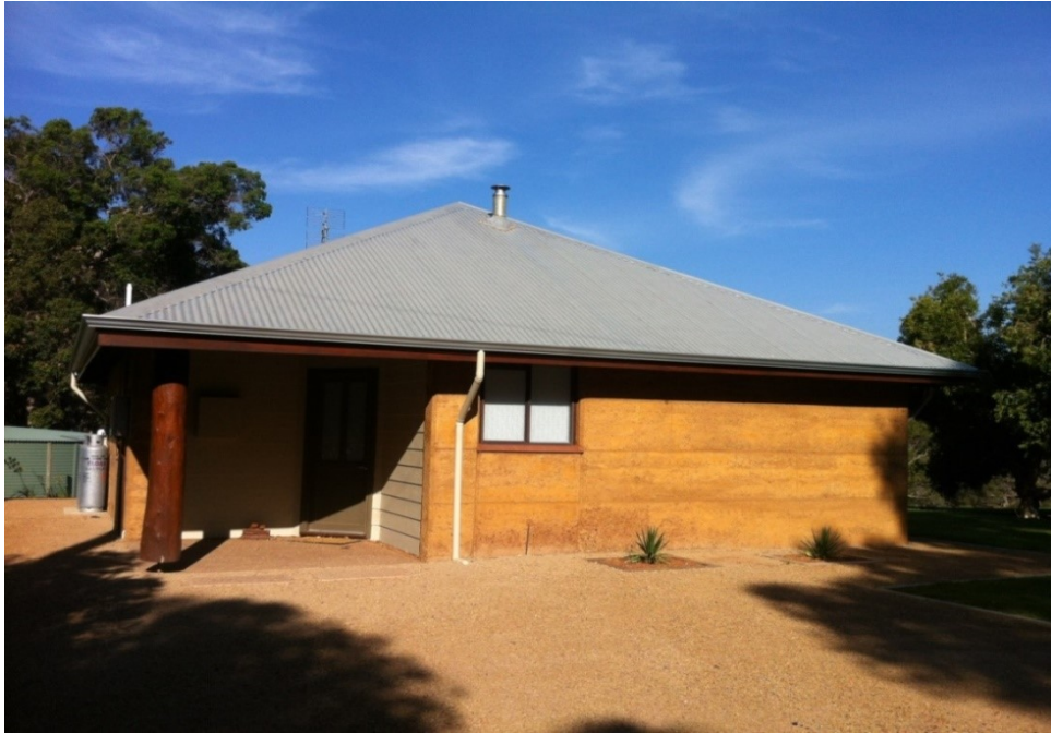
Figure 1.18 Stabilized Rammed earth construction in Australia
