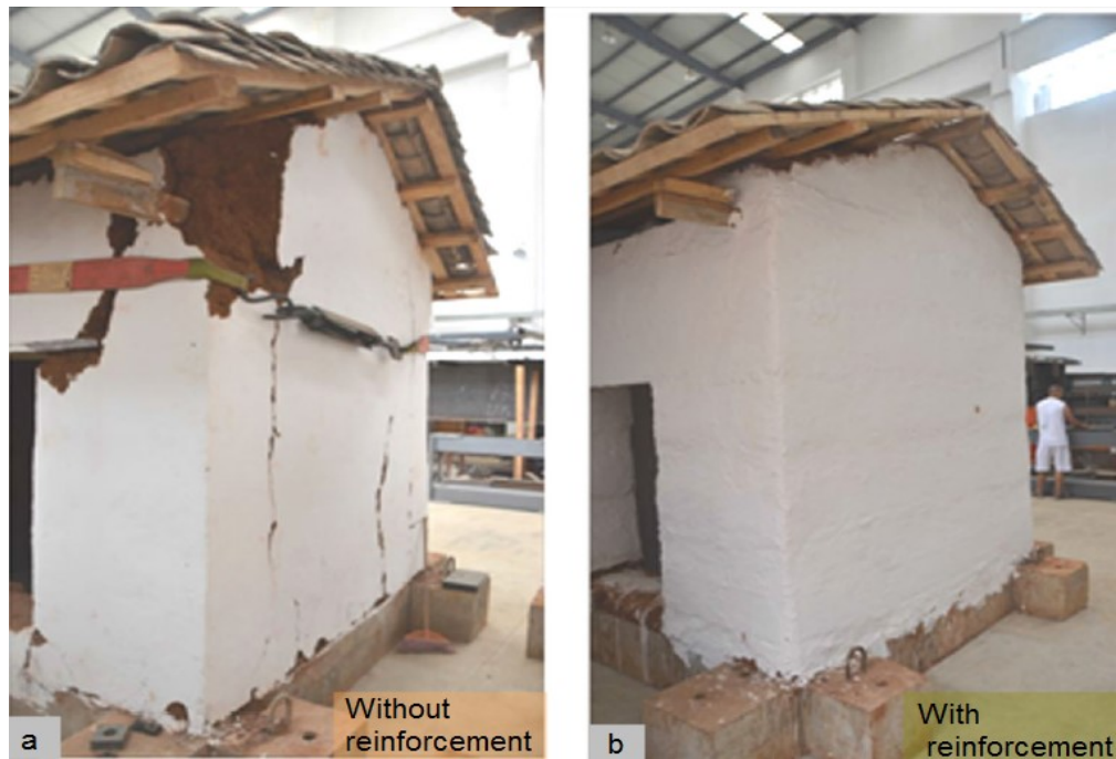
Figure A.6 Comparison of the damage between two models: (a) unreinforced model; (b)reinforced model
