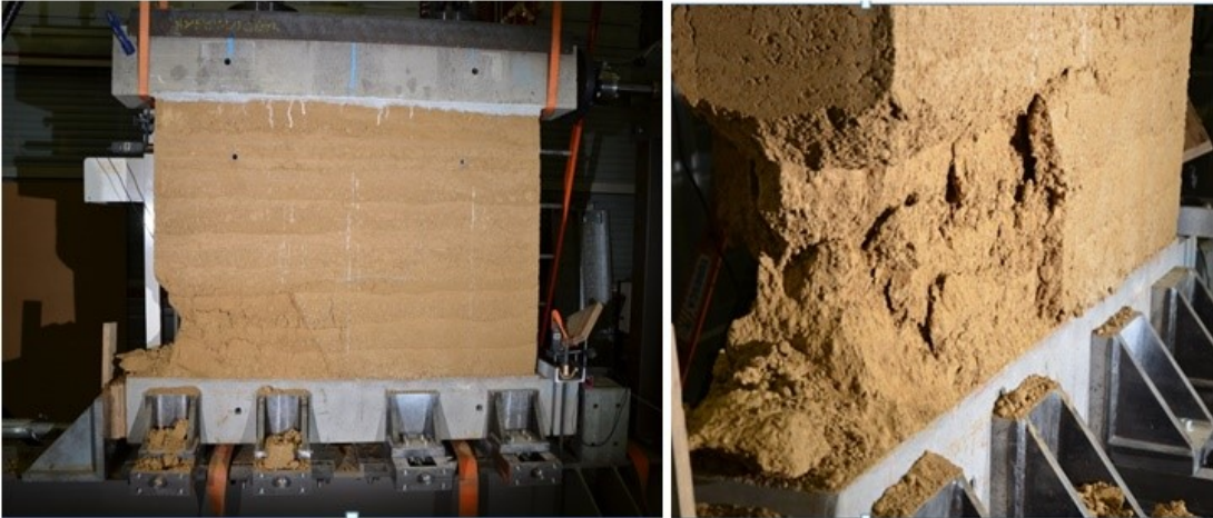
Figure 3.26 Damage of wall 1 after reaching the ultimate load
