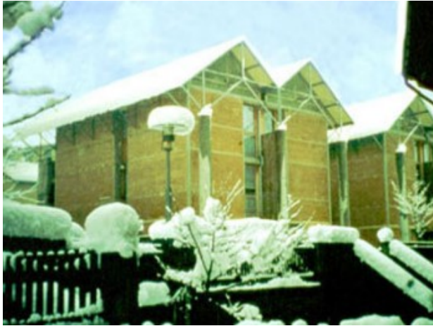
Figure 1.20 Stabilized rammed earth in Domaine de la Terre, l'Isle d'Abeau, France (from Auroville, earth institute)
