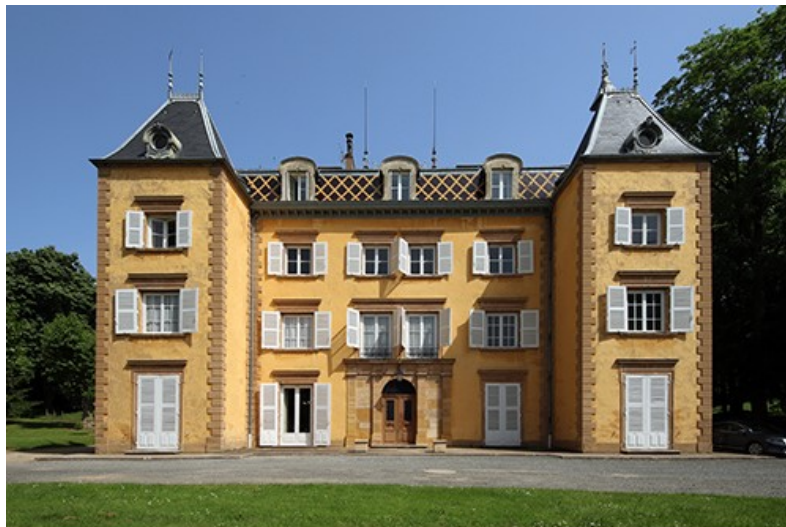
Figure 1.14 Château de Reyrieux, made from rammed earth in France, Reyrieux (Photo: Auroville, earth institute)
