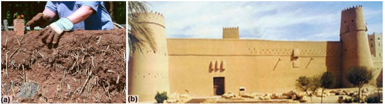
Figure 1.5 (a) Technique of Cob construction; (b) Masmak Castle in Riyadh, Saudi Arabia (Photo: M. Abdulaziz)
