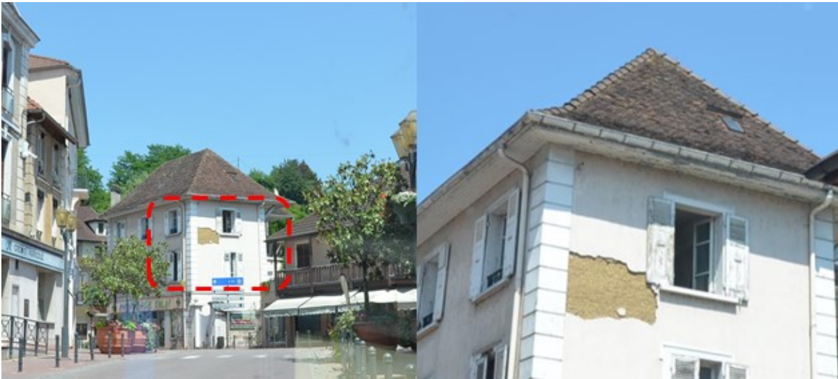
Figure 1.16 Rammed earth house plastered in “Pont de beaux voisins”, Rhône-Alpes, France
