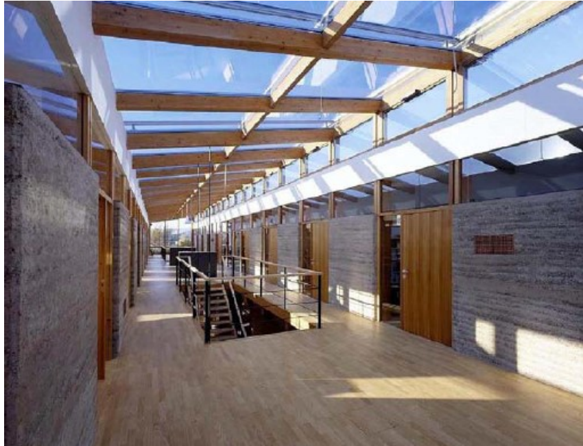
Figure 1.22 Building constructed with 160 pre-fabricated elements [22]
