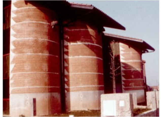
Figure 1.20 Stabilized rammed earth in Domaine de la Terre, l'Isle d'Abeau, France (from Auroville, earth institute)
