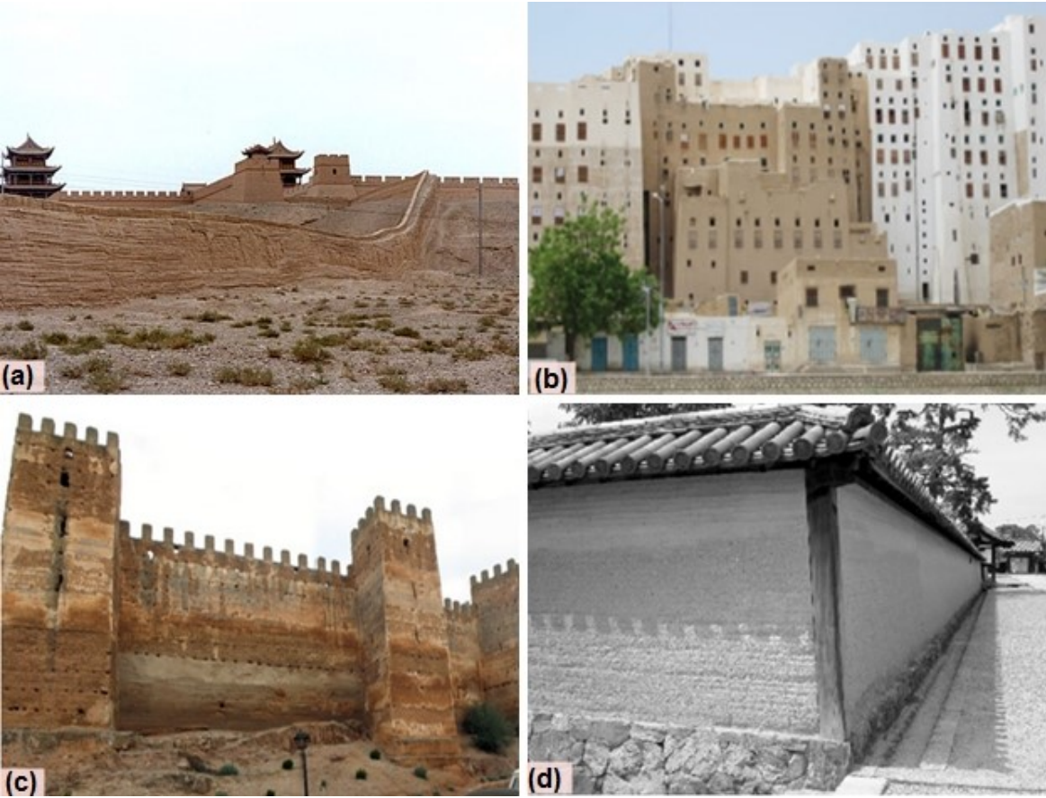
Figure 1.12 Examples of historical constructions around the world made from rammed earth: (a) Great wall of China; (b) Buildings in Shibam, Yemen (Photo: Auroville earth institute); (c) Alhambra Palace of Granda, Spain [13]; (d) Temple in Japan [12]
