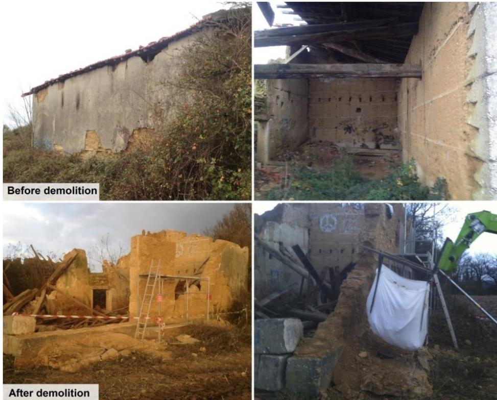
**Figure 2.6 Rammed earth soil origin: farmhouse before and during the demolition, (Photo: N. Meunier)**
