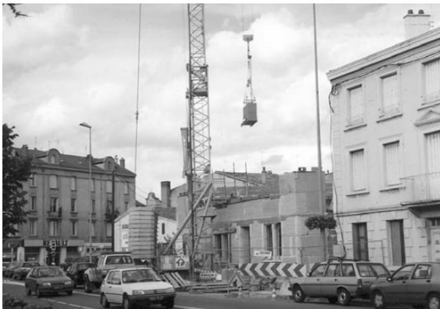
**Figure 1.21 Pre-fabricated walls being craned into position during construction at Montbrison, Loire (Photo: N. Meunier, 1995)**
