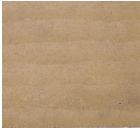
**Figure 1.11 Visible compacted layers with different thickness of a rammed earth wall constructed in the LOCIE laboratory**
