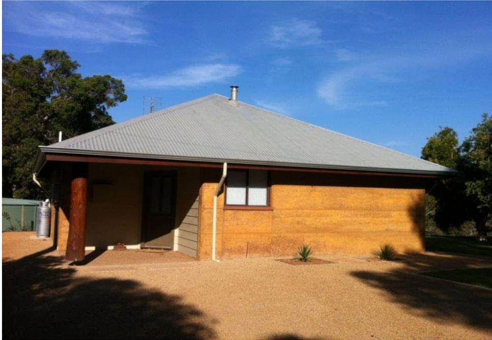
**Figure 1.18 Stabilized Rammed earth construction in Australia**
