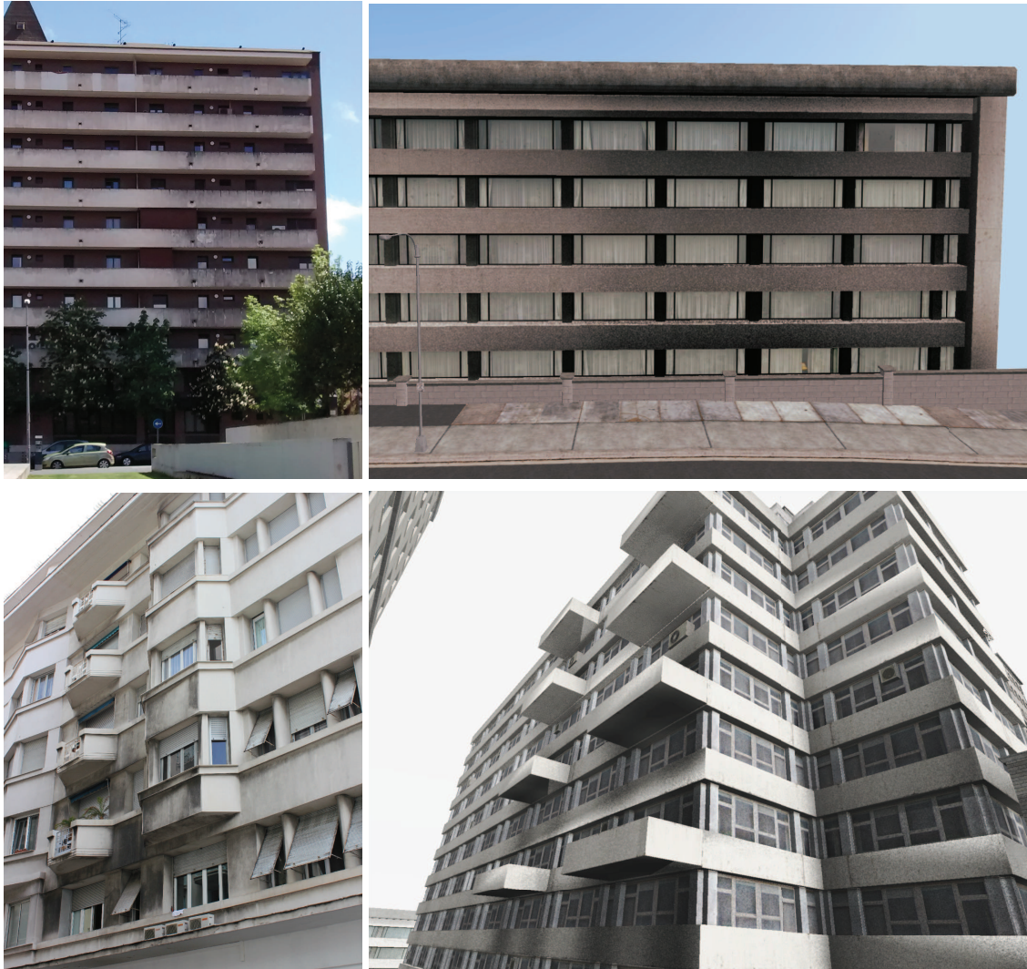
Figure IV.16: Our technique (right) is able to reproduce the behavior of real life pollution weathering effects (left). Pollution distribution and modified material appearance are comparable in a very plausible way.
