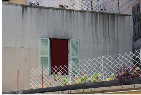
Figure IV.20: Example of deposition patterns produced by on-surface water flows.
