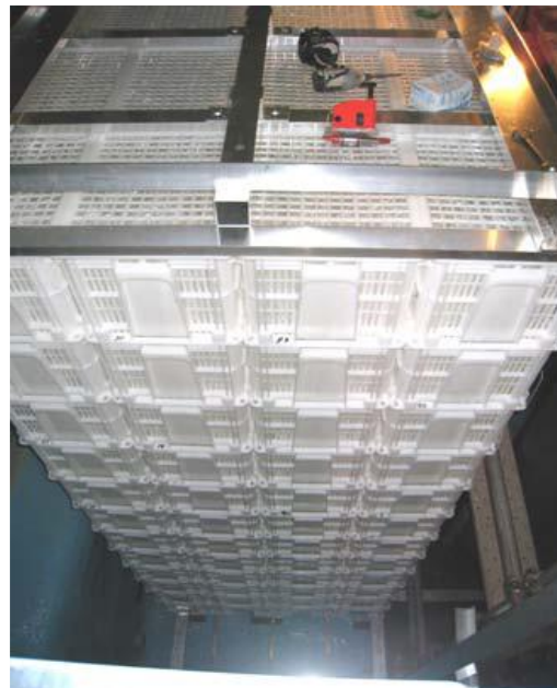
Figure 3.4 - Typical installation of the plastic cases into every isolated tank.
