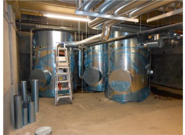
Figure 2. 24 - Water tanks used as heat storage before (left) and after (right) full insulation.
