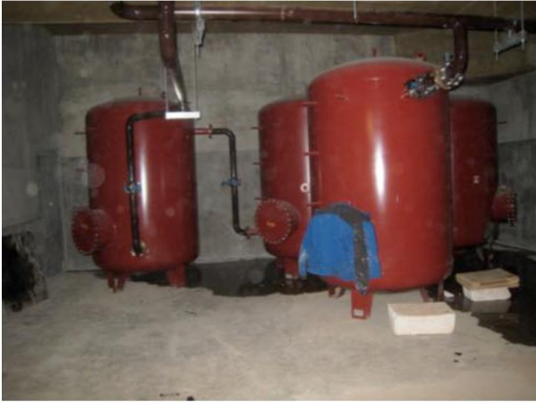
Figure 2. 24 - Water tanks used as heat storage before (left) and after (right) full insulation.
