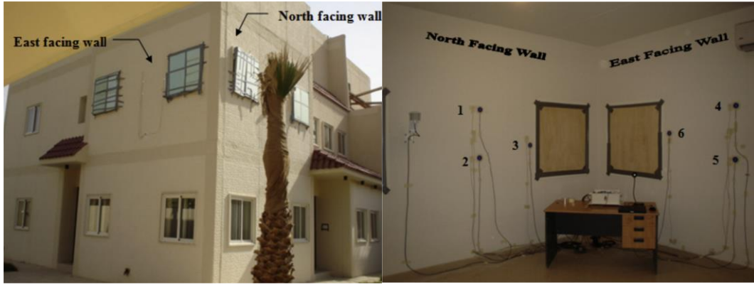
Fig. 1-10 The instrumented building and the test room walls [21]
