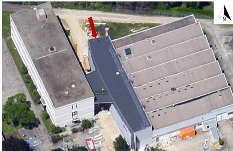
Fig. 2-21 A demonstration building-Platform SYNERGI
