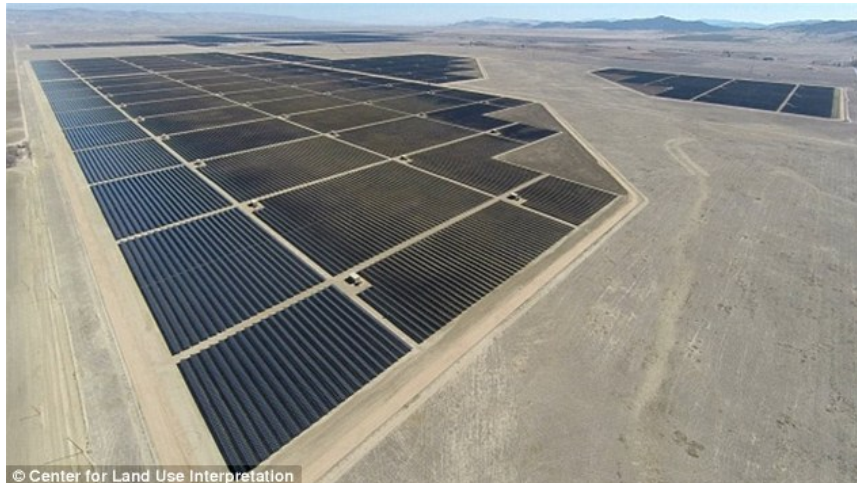
FIGURE 1.2: the Topaz solar farm.
