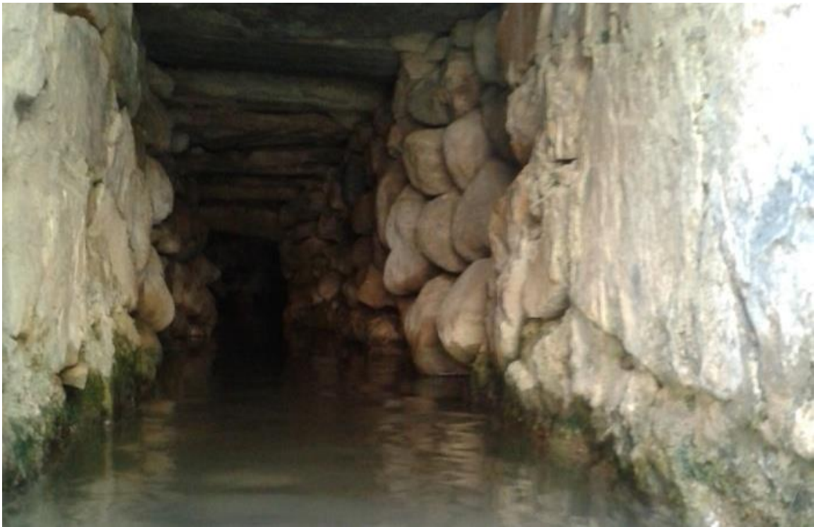
Karez, a popular traditional way to abstract and convey the water, Shakar Dara, Afghanistan (Field survey 2013)
