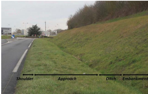
Figure 1. A general scheme of zonation of the road verges (sensu Frenkel 1977). The approach zone was used for vegetation sampling in north-west France.
