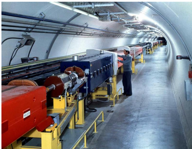
Figure 1.5: View of the SPS tunnel.
