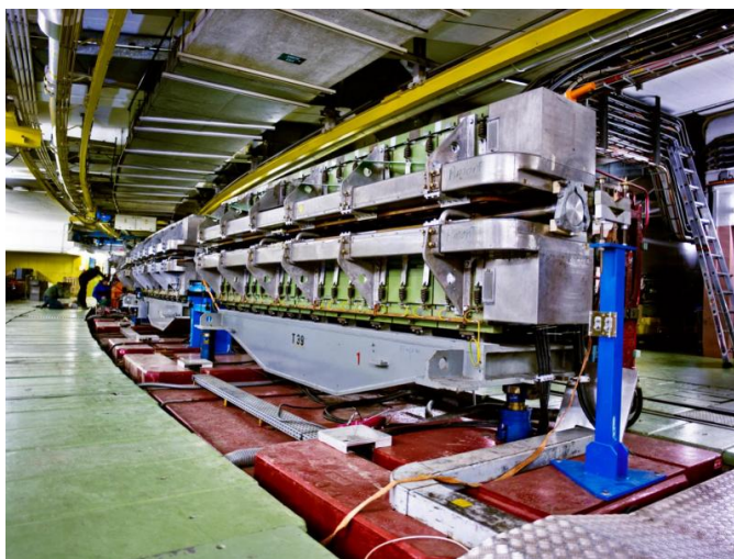
Figure 1.4: A section of the PS during maintenance.
