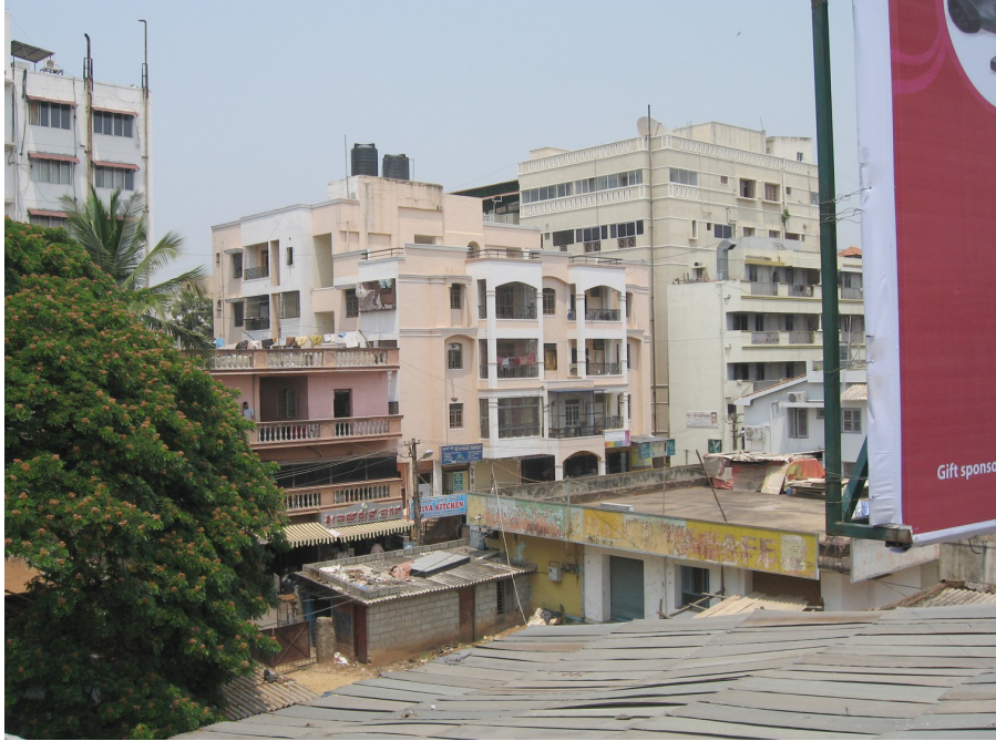
(a) Près de Domlur, HAL Airport road, Bangalore.
