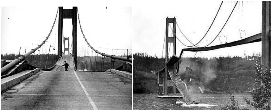
Figure I.1: Endommagement et rupture du pont Tacoma (Billah et al. 1991)
