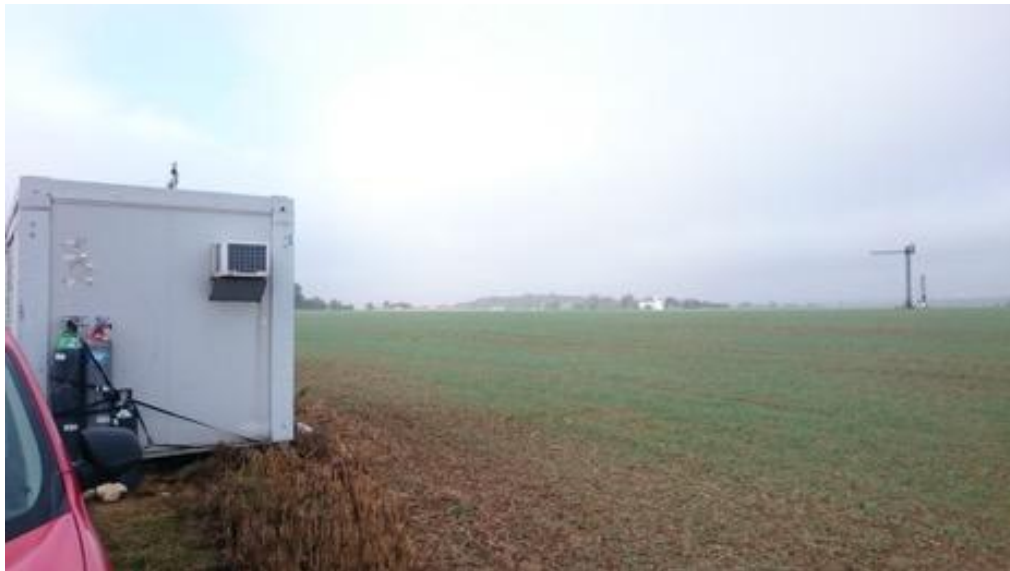
Image 4-3 To the left, the building within which the CRDS, and GCs are located during the two long-term measurement campaigns. Instrument inlets are co-located on the roof of the building. The meteo-station and flux tower can be seen on the right-hand side of the image.
