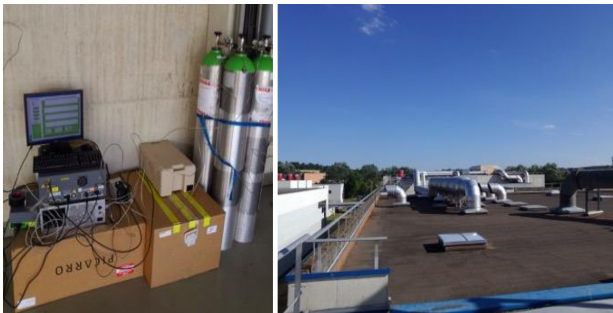
Image 4-6 : (Left) Set-up of CRDS instrument with calibration and target gases located within the filtration building. (Right) location of inlet on the roof of the building, image faces north.
