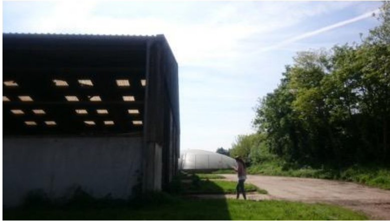
Image 4-1 Sources are located within close proximity. Dairy Barn, housing containing lactating cows to the left, and the Biogas production unit in the background.
