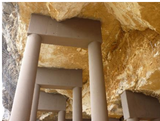
Figure 2-12 Supporting structures inside the cavern
