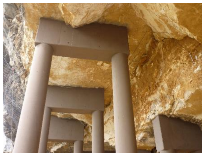
Figure 2-12 Supporting structures inside the cavern
