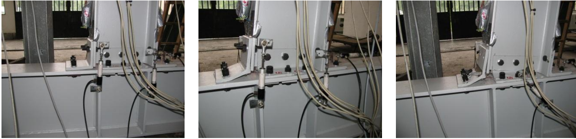
Figure 5.14 Deformation of connection elements during experimental testing
