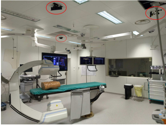
(a) Positions of the ceiling-mounted RGBD cameras installed at an experimental interventional room at IHU Strasbourg marked in red.
