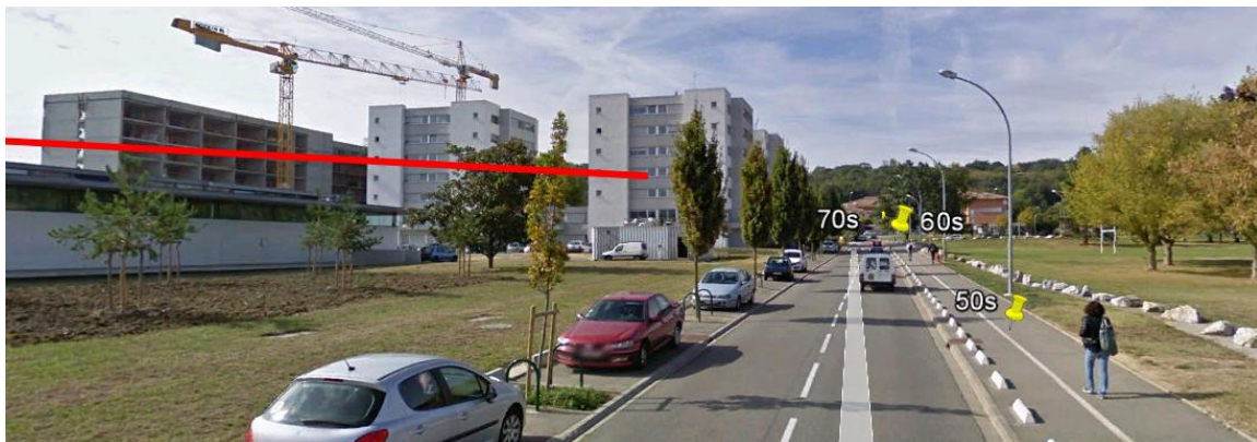
Figure 5.8: Building causing strong multipathes
