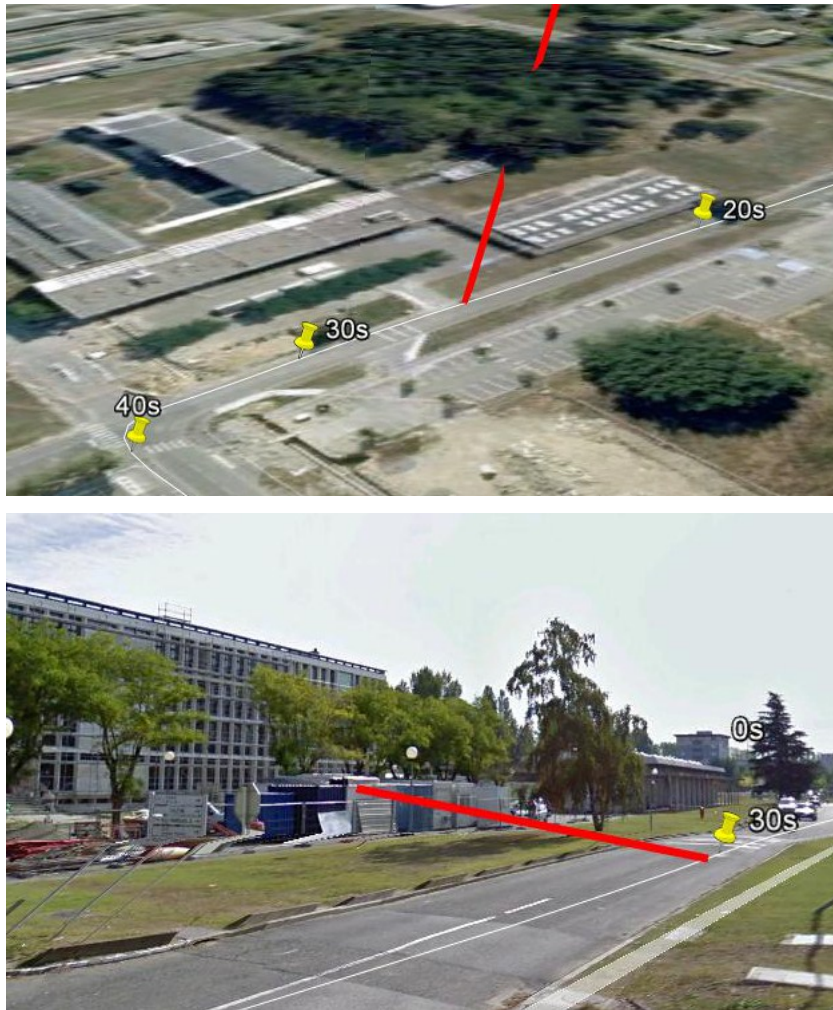
Figure 5.7: Buildings causing the attenuation of the direct signal
