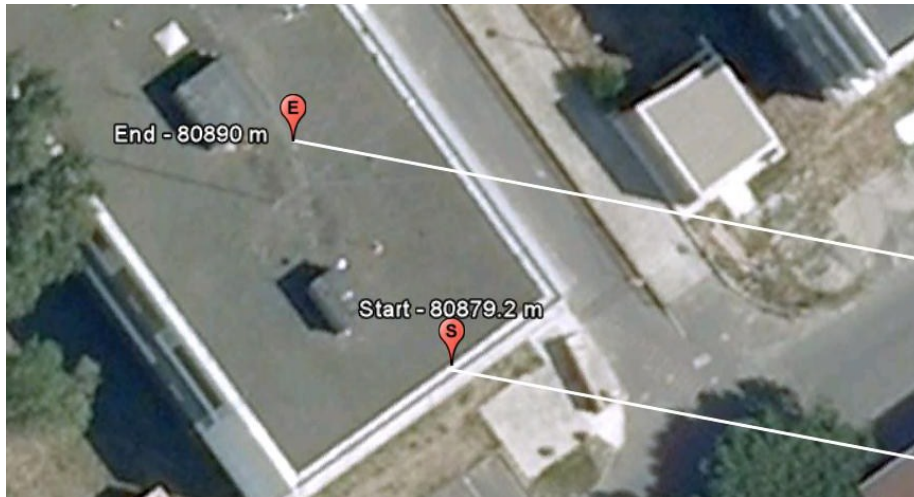
Figure 5.17: Sat. view of the test configuration
