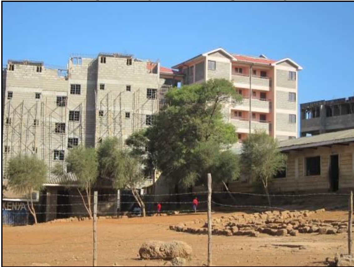
Plate 3. 3: Partially complete housing unit next to a complete housing unit
