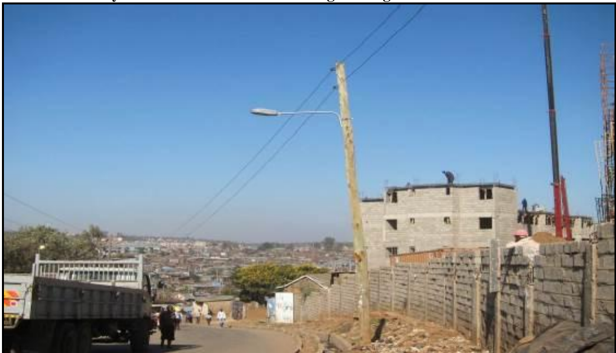
Plate 3. 2: Partially constructed houses overlooking the original slum houses
