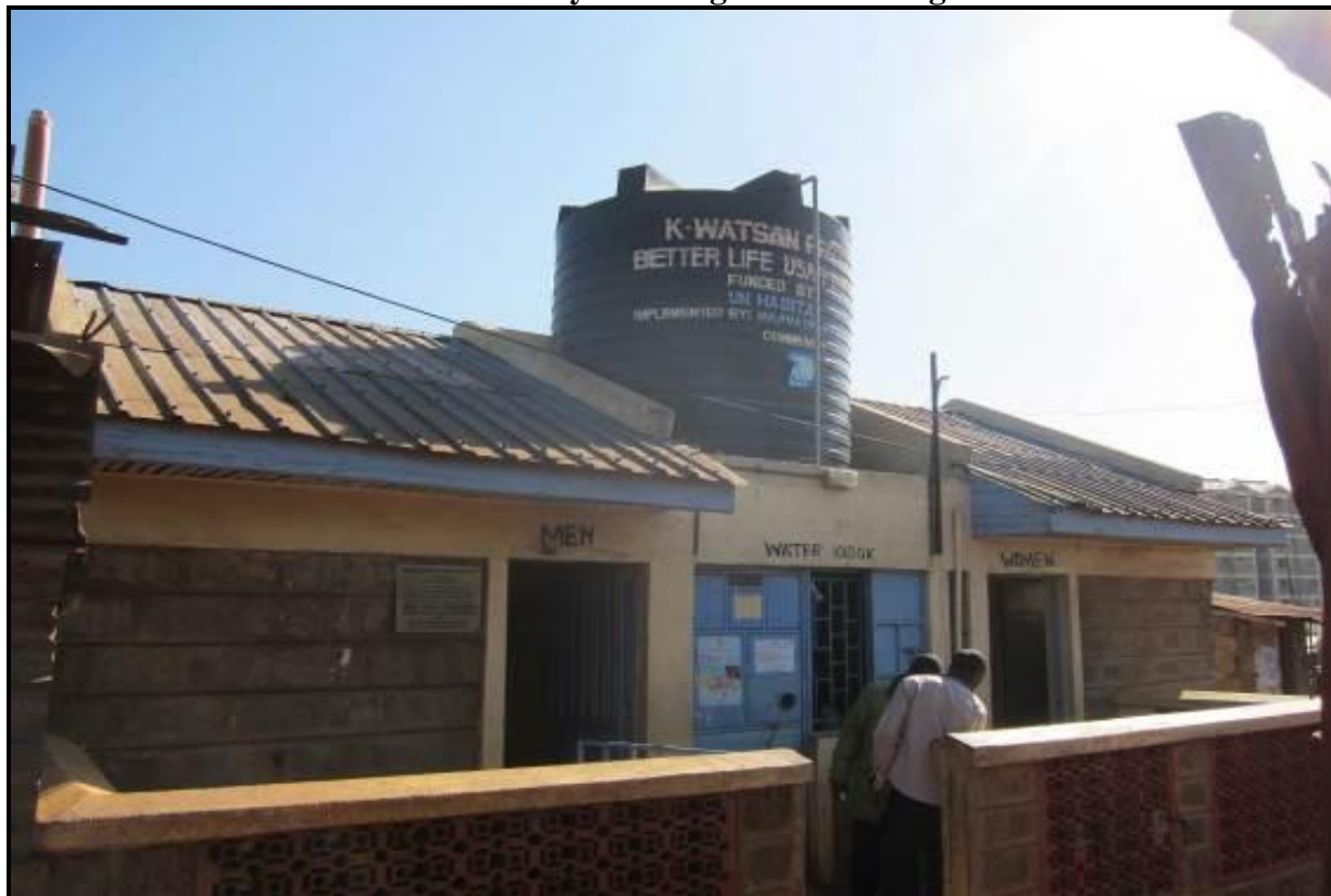
Plate 3. 1:K-WATSAN sanitation facility towering over the village
