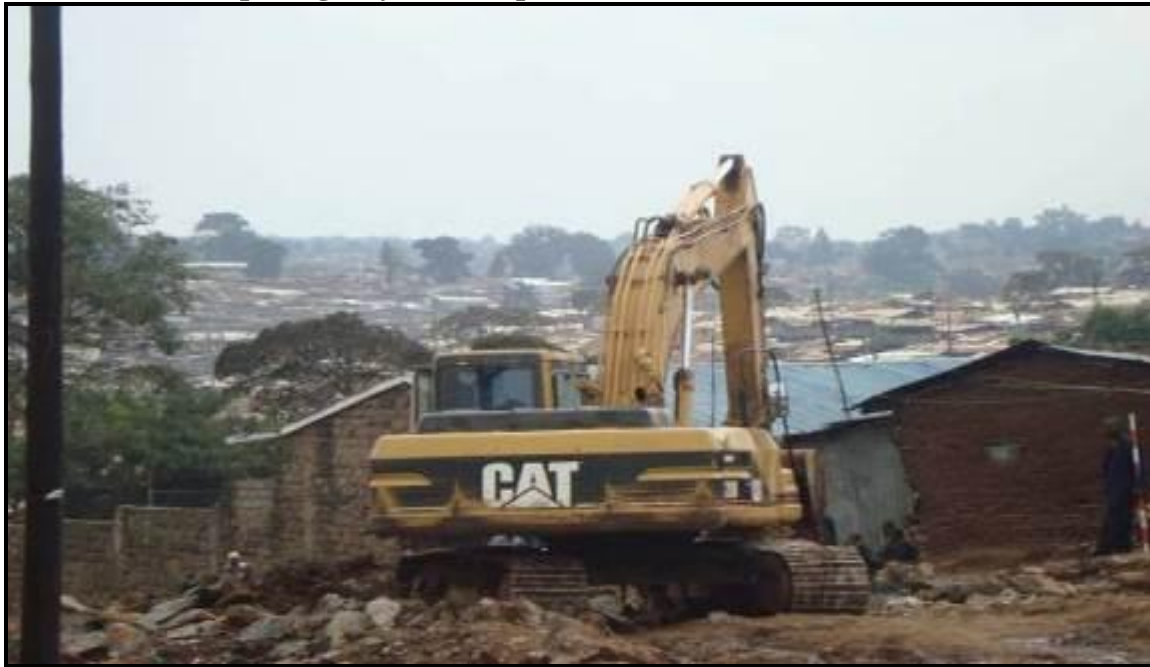
Plate 4. 3: Tractor paving way for the spine road
