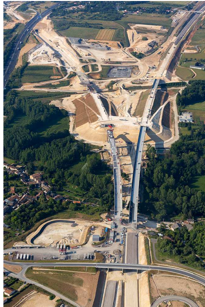
Figure 2.3: Aerial view of part of a stretch of the SEA line; source: Vinci Construction Terrassement
