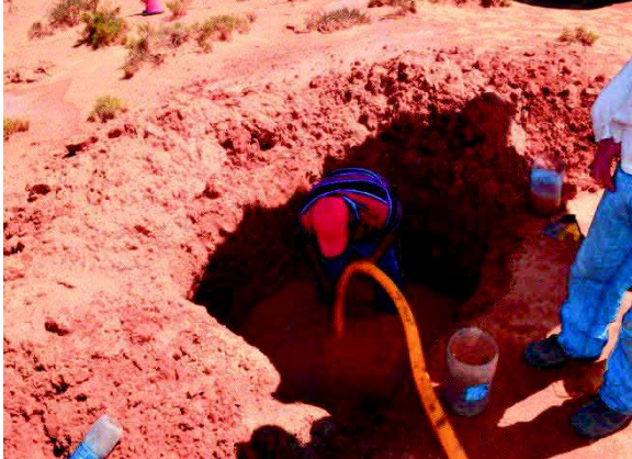
Fig. 39: Pumping machine to discharge the underground water.
