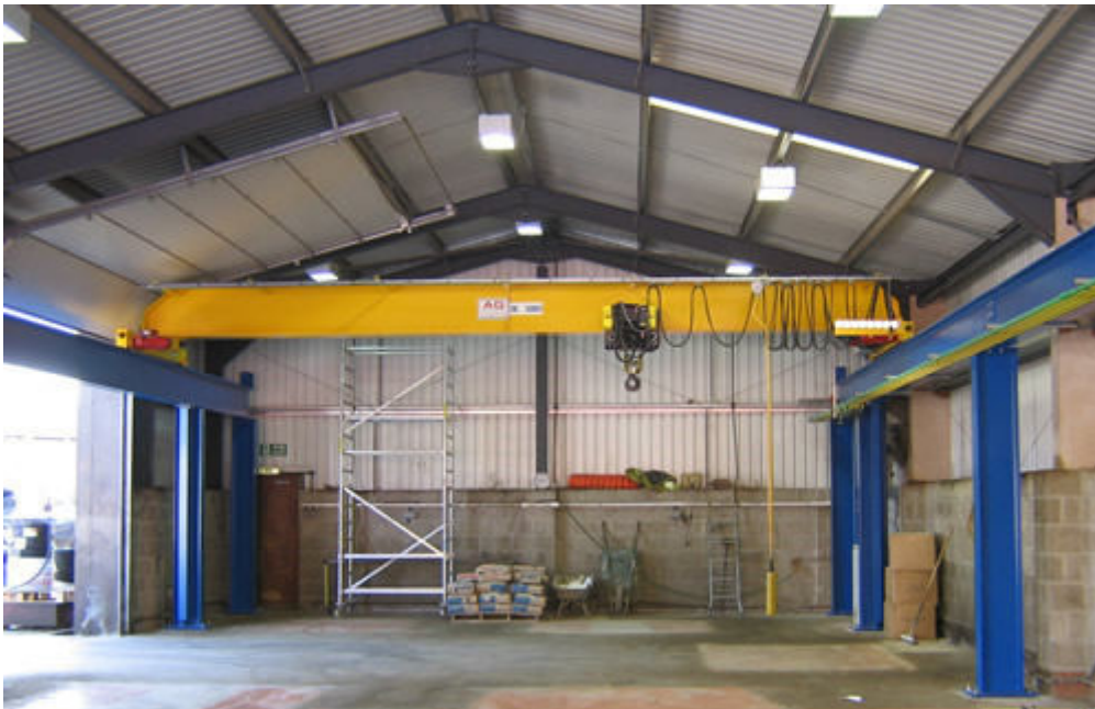
Figure 1-1: Example of a crane girder
