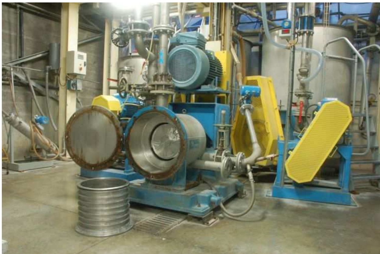
Image 1: General view of the pilot plant screening facility
