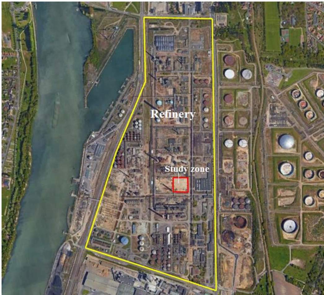
Figure 7.1: The location of the study zone (Google Earth). The study zone is located in the center of the refinery and covers an area of around 5600 m 2 .
