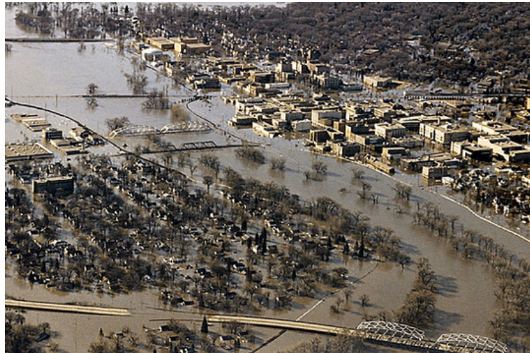
Figure 2.7 – Grand Forks after levee over-topped.
