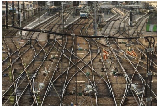
Figure 1.1 Railway track next to Gare d'Austerlitz in Paris.
