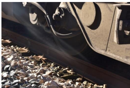
Figure 1.3 Ballast surrounding the sleepers below the rail.
