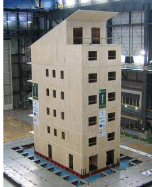
(b) Seven Storey X-Lam Building
