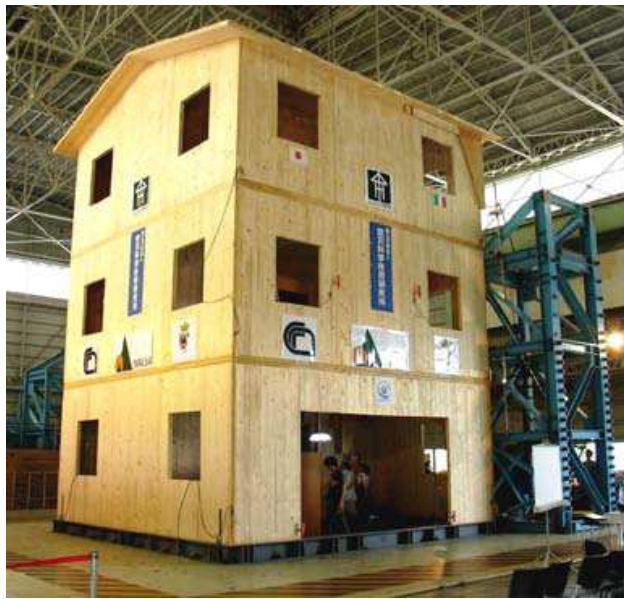
(a) Three Storey X-Lam Building
