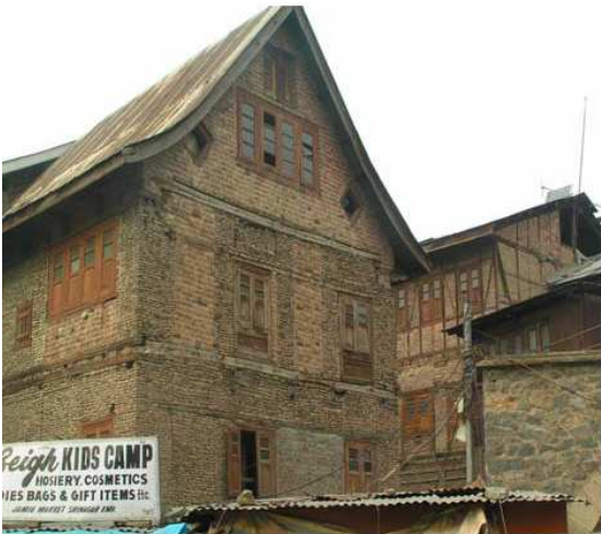
Fig. 2.4: Sample of Taq structural system.[124]
