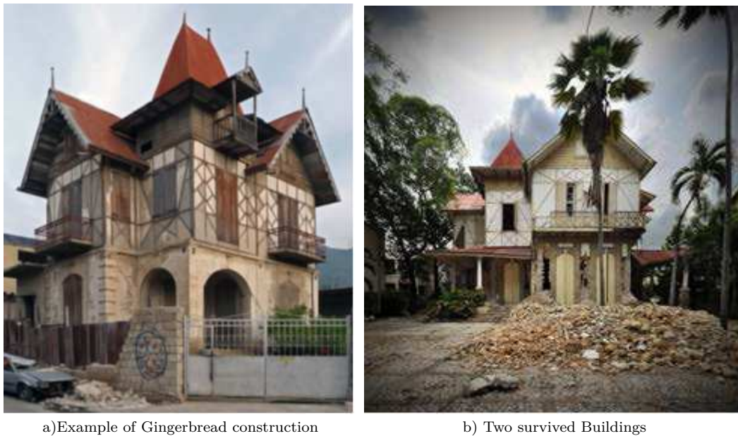
Fig. 2.9: Gingerbread Structure in Haiti [16]
