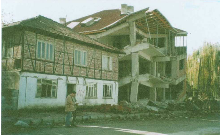
Fig. 1.1: Two adjacent buildings concrete and traditional timber in Turkey, [48]
