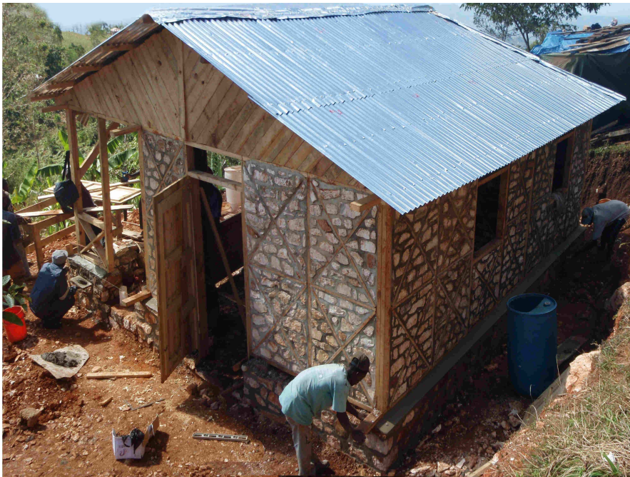
a) Enhanced Sample of Kay Wall [85].
