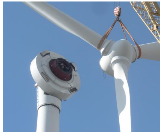
b. Installation du prototype
