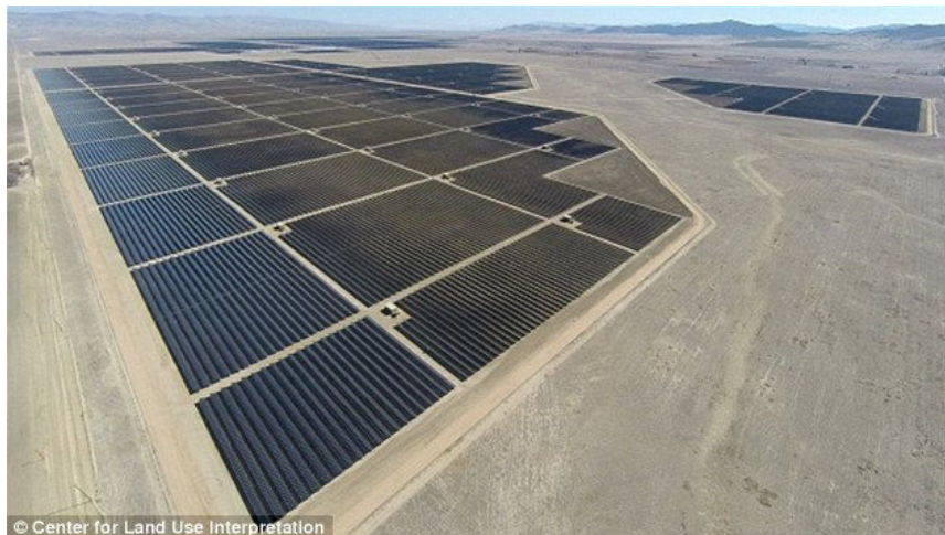
FIGURE 1.2: the Topaz solar farm.
