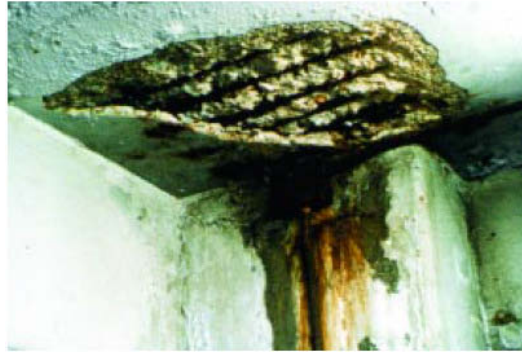
Figure 3.1: Corrosion of reinforcing steel.
