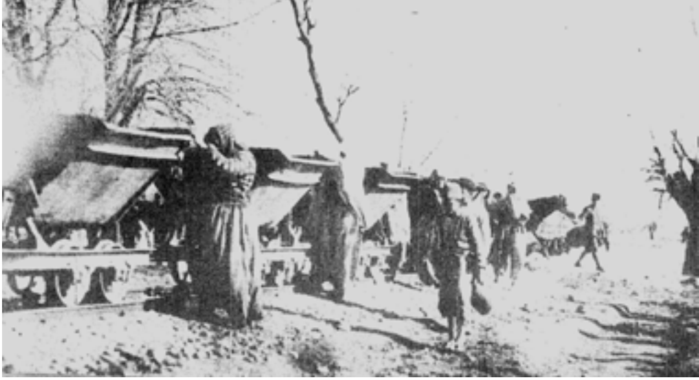
Fig. 27 Women working on the Azarköy railway during the National Struggle.
